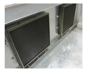
Steel square matrix 10 mm x 50mm used to form WGBC for air ventilation
